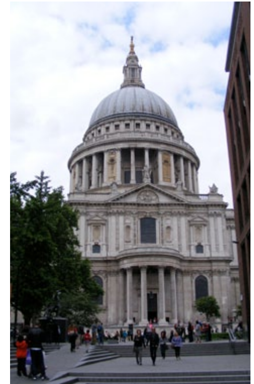
Christopher Wren used Portland Stone for the construction of St Paul's Cathedral in London.
