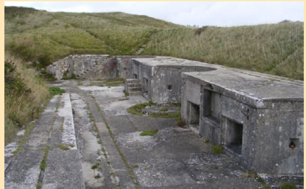
The remains of the Victorian High Angle Battery.
